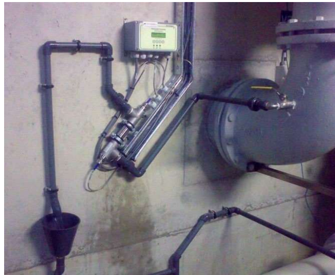
Final installation of a Kemtrak DCP007 photometer
